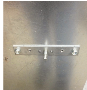
Factory installed anti-rotation bracket. Remove and disregard.
