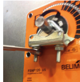
Loosen using a 10mm wrench or socket.
